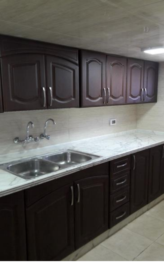
Rehabilitation Mneen Health Center ( Medair)
