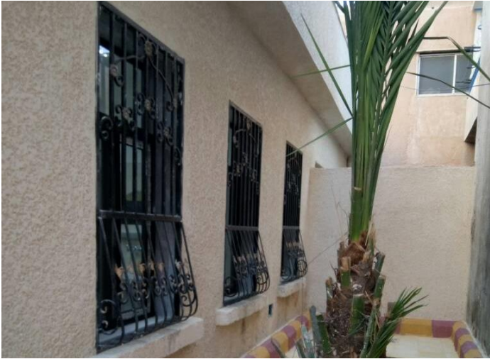
Metal work- Rehabilitation Mneen Health Center ( Medair)
