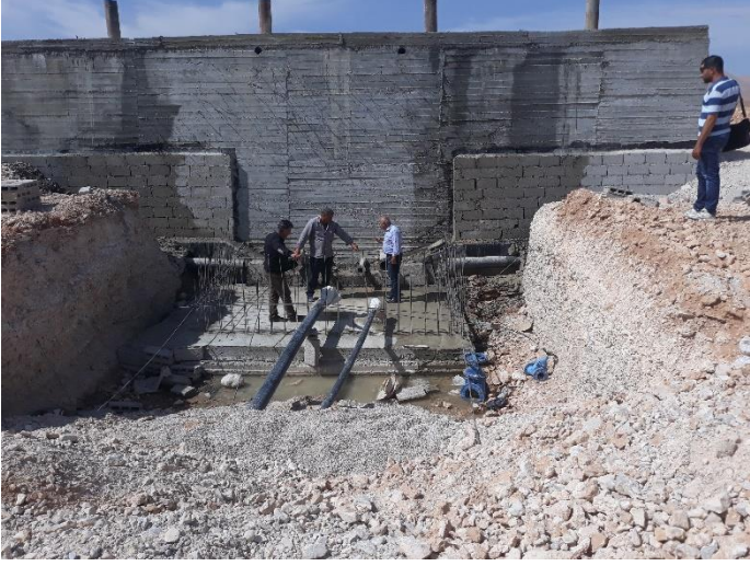
WASH (Construction of Irrigation System in Qara- Rural Damascus) / (AAH)
