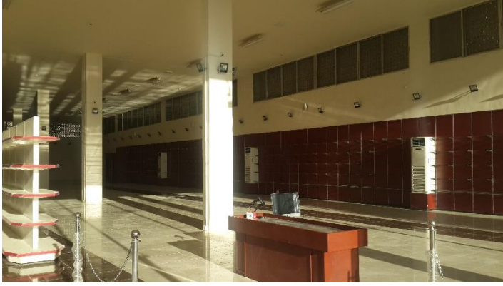
Mall (Rehabilitation works of JARAMANA Mall)
