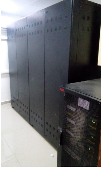
UPS (Provision of Rehabilitation Works at Children Hospital in Damascus) / (WHO)
