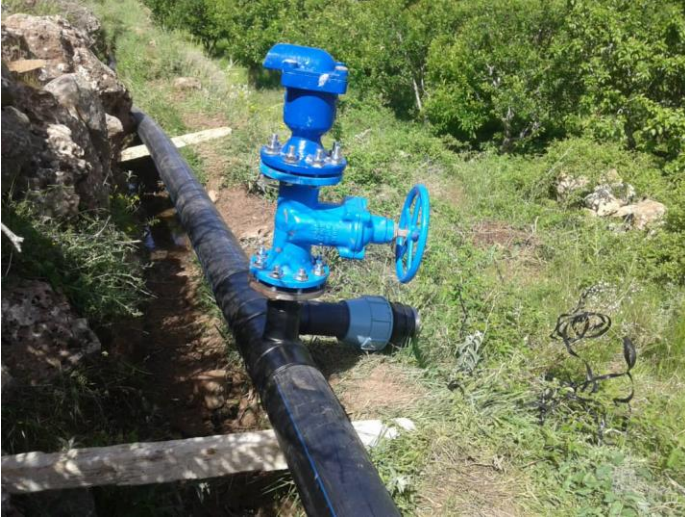
Rehabilitation of Main Irrigation Canal in Arna Area - Rural-Damascus/ (AAH)
