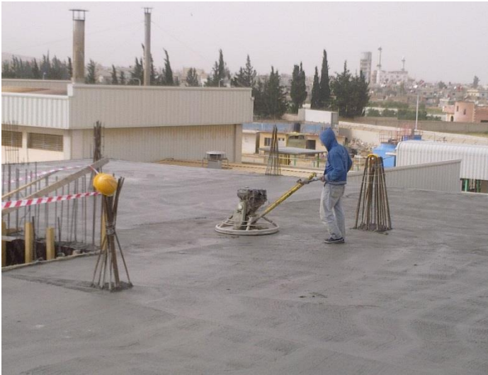
Concrete works (THE EXTENSION BUILDING AT NESTLE SYRIA)
